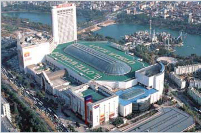
Four ORE-300XL units and one ORE-400XL unit provide partial cooling for this multi-purpose business complex in Seoul, South Korea.
