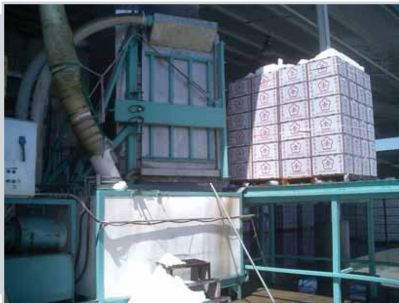
An ORE-100 is used to produce packaged ice that is injected into boxes of broccoli for cooling during transportation.
