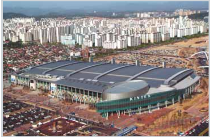
Korea International Exhibition Center in South Korea is cooled with four ORE-300XL units.
